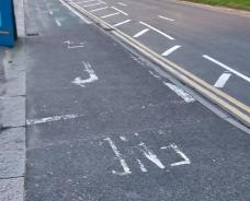
Additionally, the existing green high friction surface treatment is almost gone from cycle track from Chalkwell Avenue to Western Esplanade. It will cost in the region of £210,000 to re-apply the green high friction surface treatment on the cycle track from Chalkwell Avenue to Western Esplanade.
